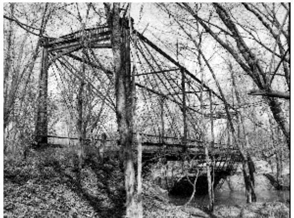
The historic Fink Truss Bridge, which spans the Connotton Creek, is now part of Camp Tuscazoar.
