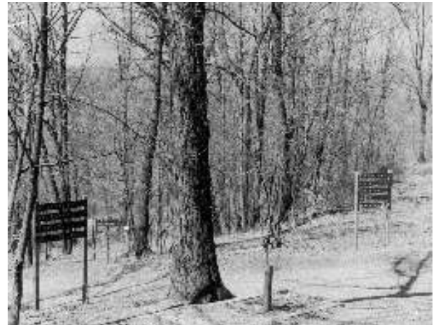
Brian Harmon constructed and installed new campsite directory and traffic direction signs.
