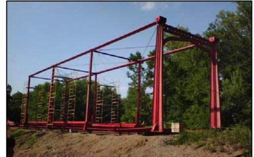
*The Zoarville Station Bridge is being re-assembled and will be lifted into position.*
