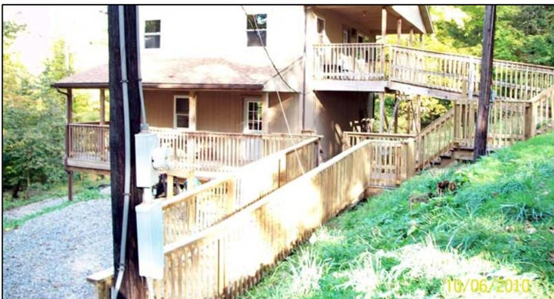
*Photo of completed decks, stairs, railings and ramp at the recently-completed Richard W. Belcher Memorial Lodge.*
